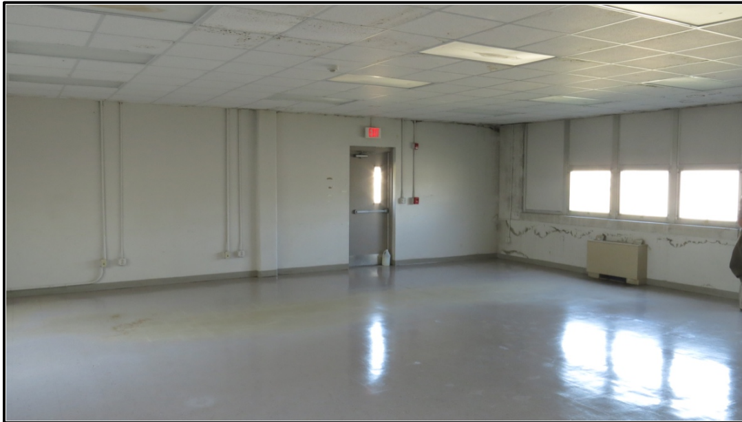
Figure 7. Classroom area inside Bldg. 6733.
