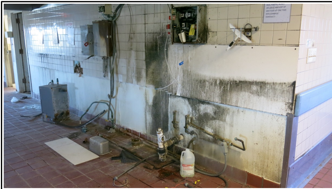
Figure 4. Kitchen area inside Bldg. 2261.
