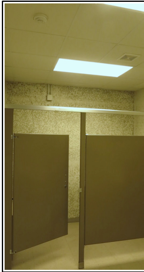
Figure 8. Bathroom area inside Bldg. 6733.
