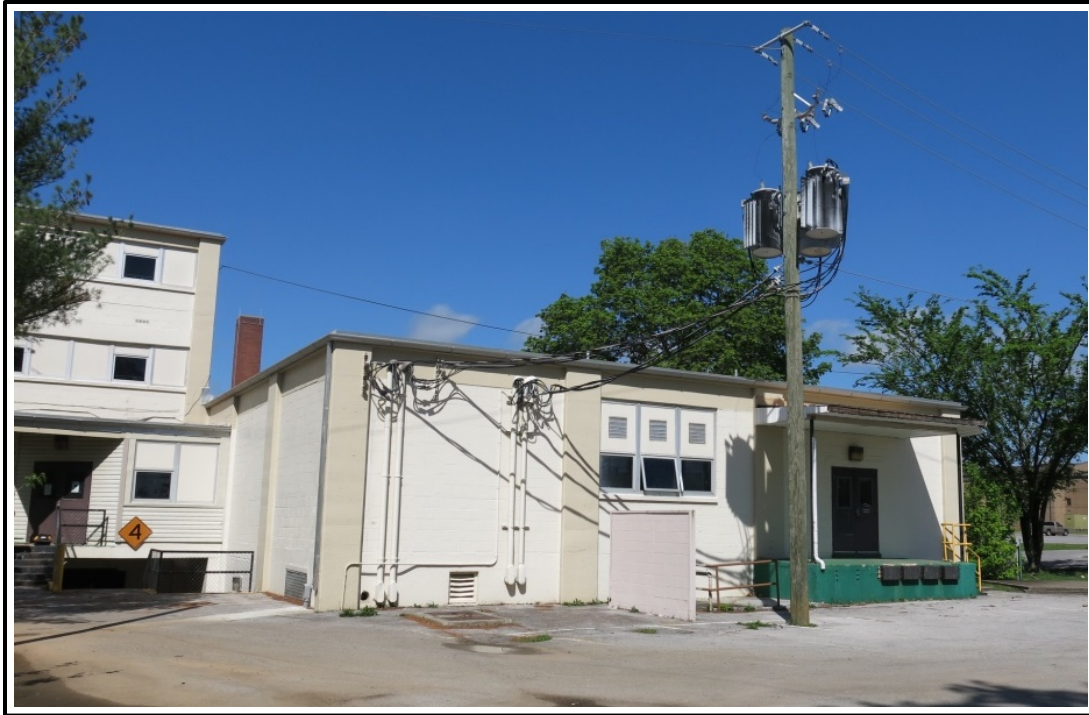
Figure 6. Exterior of Bldg. 6733 – barracks.
