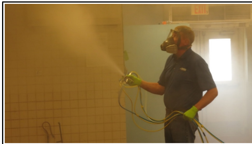
Figure 14. Dry-fog being applied to intake of HVAC ducting Bldg. 2261.
