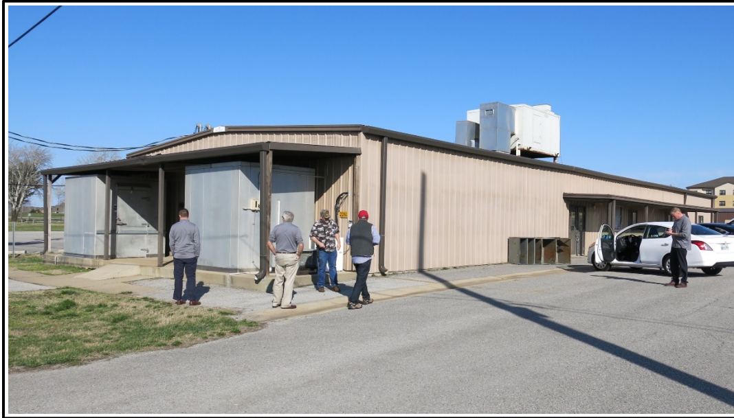
Figure 3. Exterior of Bldg. 2261—dining facility.
